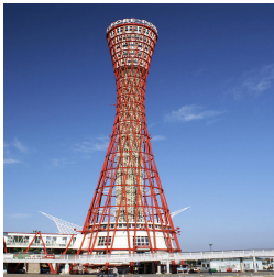
Kobe Port Tower
