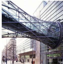
Corp o Street Bridge
